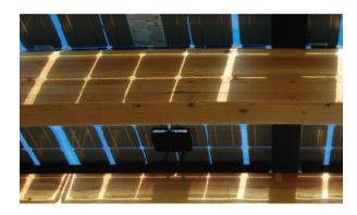
Often referred to as Glass on Glass units, the smaller gaps between the PV cells provide the shading while still allowing a substantial amount of natural light to filter through and radiate the space underneath.
