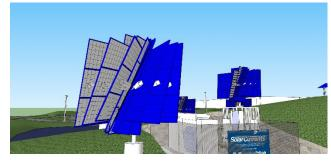
The solar array is made up of 25 rows of panels paired with seven dual axis trackers that will rotate the panels to align with the sun as it moves during the day.
